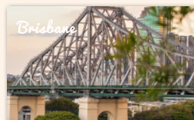
Story Bridge Adventure Climb
